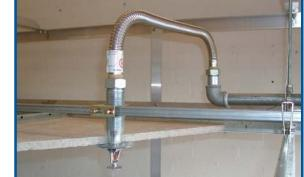
Rapidrop® is a complete unit, a corrugated stainless steel flexible with nipple, reducer, bar and brackets, which are fitted to the ceiling tile support rails to locate and secure the sprinkler in the correct position. As well as considerably reduced installation time, the risk of mess (from the cutting and threading activity associated with the traditional armover method) in the clean area below the suspended ceiling is eliminated, allowing other activities to proceed more efficiently.
